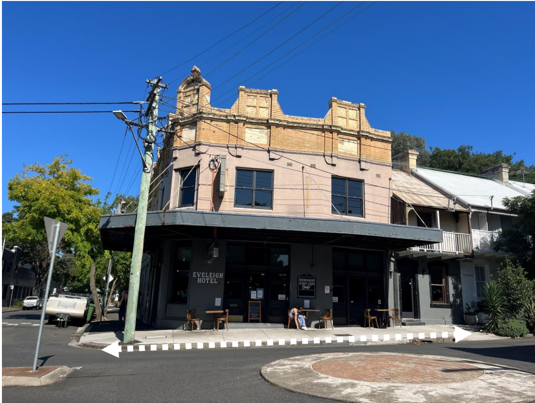
Figure 3: Site viewed from Abercrombie Street
