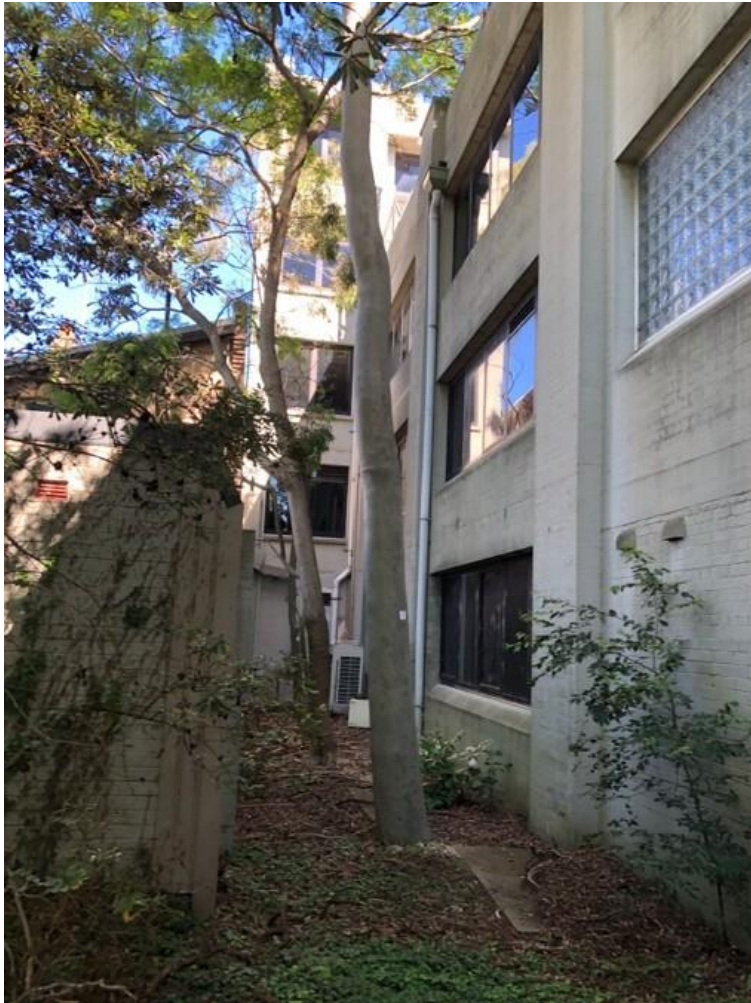
Figure 9: View along rear southern boundary
