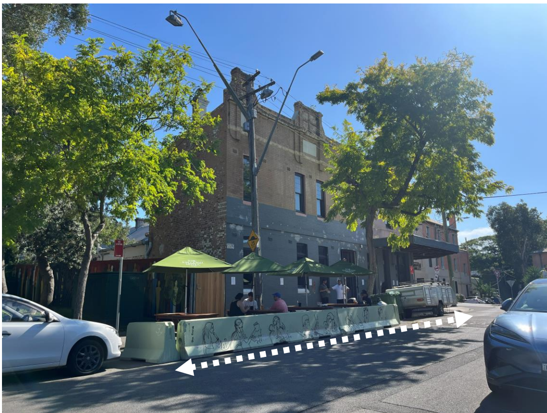
Figure 4: Site viewed from Vine Street
