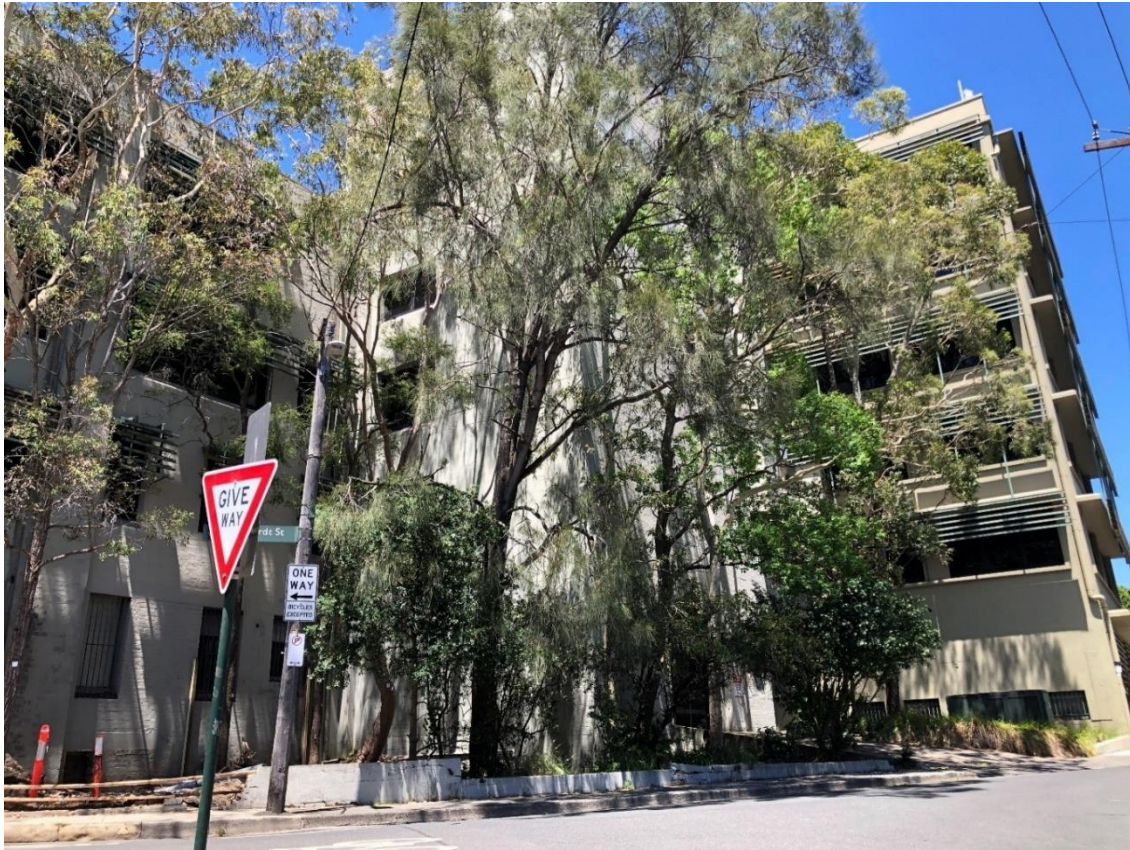
Figure 5: Site viewed from Leichhardt Street looking south
