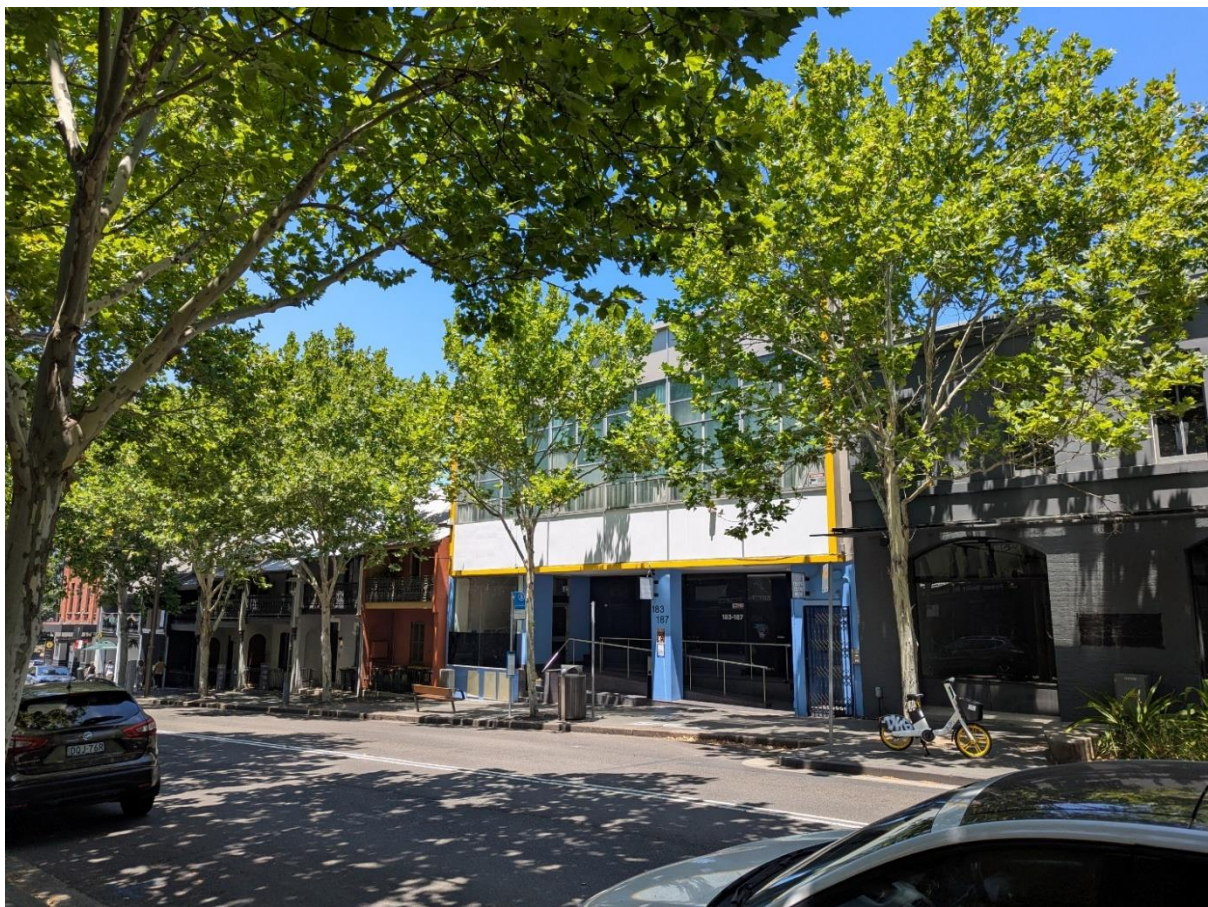
Figure 2: Site viewed from Harris Street facing west (in yellow and blue)
