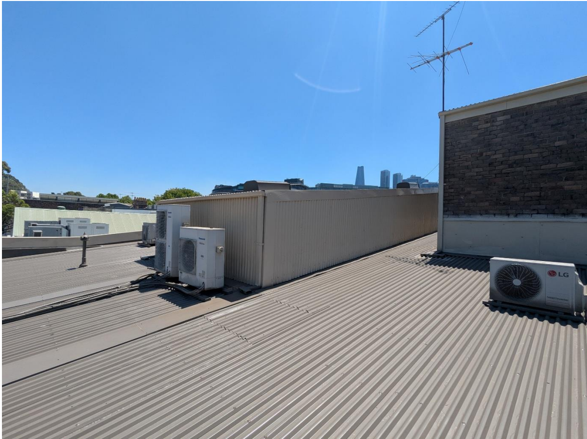
Figure 20: Photo of the existing roof looking north, showing the central non-habitable roof form (left) and lift overrun/stairs (right)
