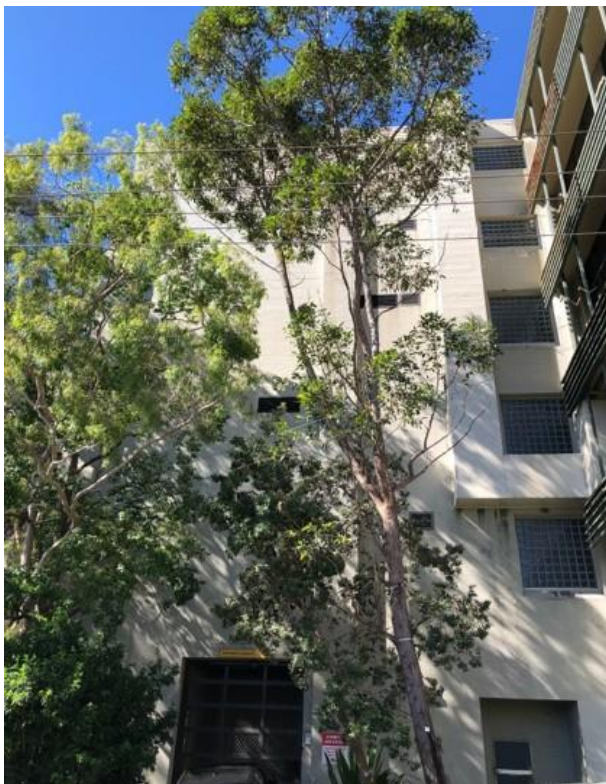
Figure 6: Site viewed from Leichhardt Street looking south
