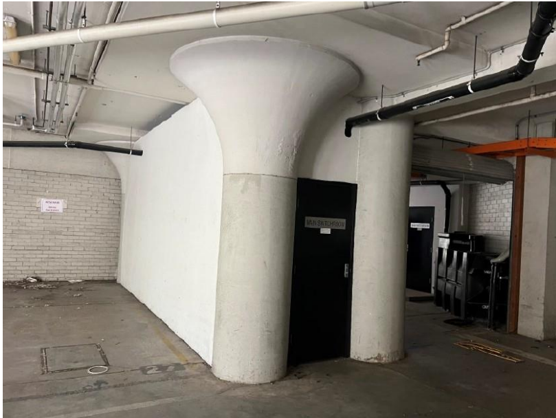
Figure 11: Mushroom column within basement
